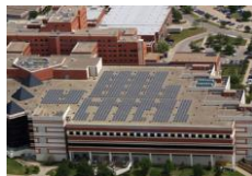
On-grid commercial/ industrial roof-tops
